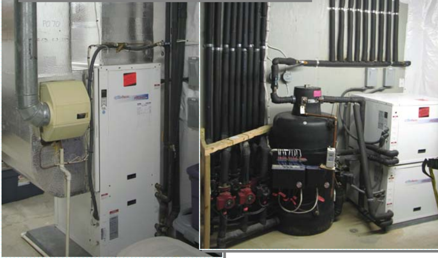
WaterFurnace heat-pumps [ Left: forced air. Right: for radiant floor ]
