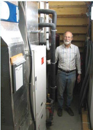
WaterFurnace heat-pumps [ Left: forced air. Right: for radiant floor ]
