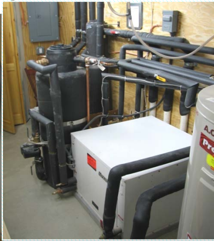
WaterFurnace heat-pumps [ Left: forced air. Right: for radiant floor ]
